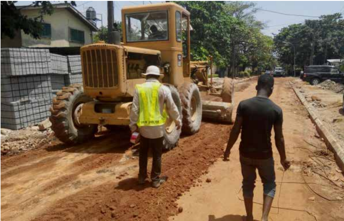
Babatunde Jose Road under construction
