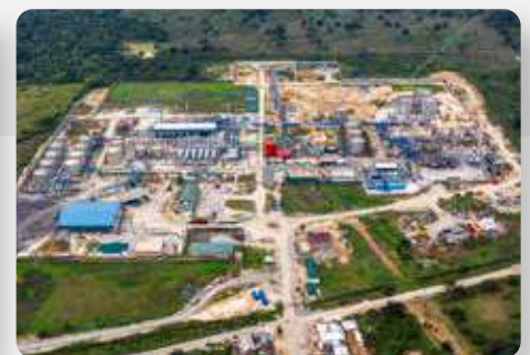
2019 Construction increased to include the completion of the Refinery Expansion Project, the Diesel Loading Bay and also storage tanks for crude and refined products.
