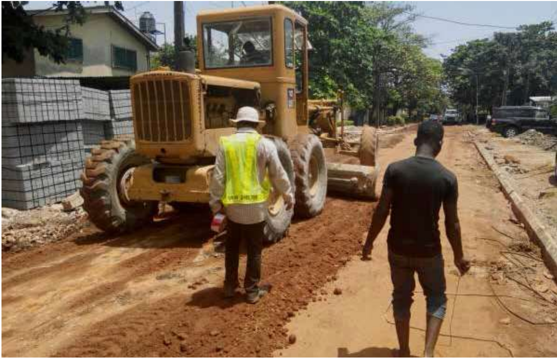
Babatunde Jose Road under construction
