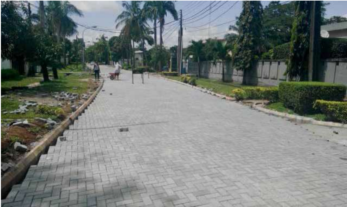
The completed Babatunde Jose Road
